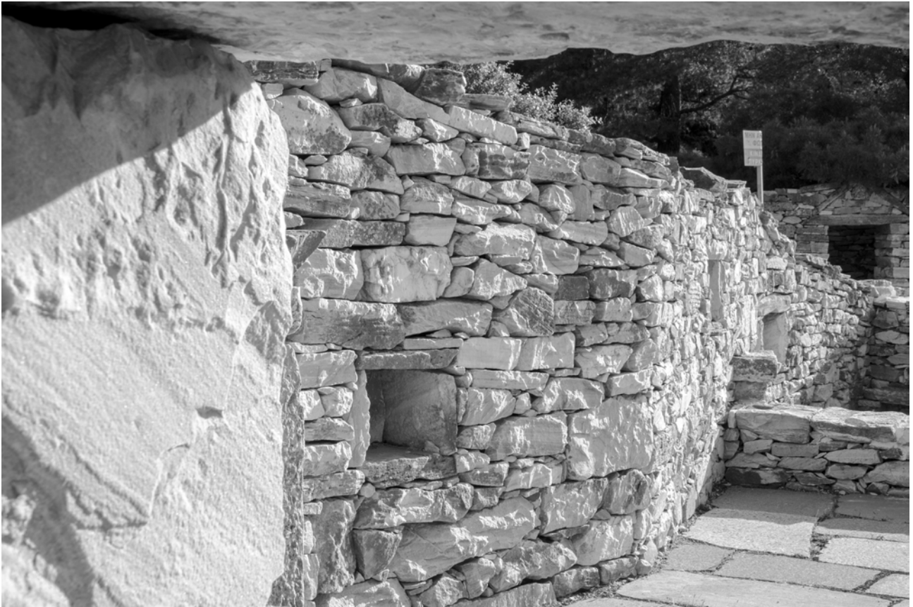
Fig. 1 Nella Golanda and Aspasia Kouzoupi (1997). Open Air Museum of Quarry Arts, Aloula, Mount Pentelicon. Restored Houses for Seasonal Workers. [Photo: Maria Mitsoula, 2018]
